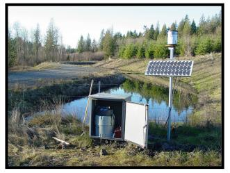
Bioswale and Infiltration Pond – increases natural seepage into the ground
