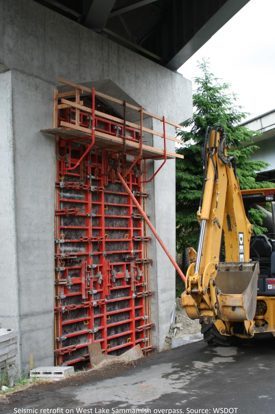
Seismic retrofit on West Lake Sammamish overpass. Source: WSDOT
