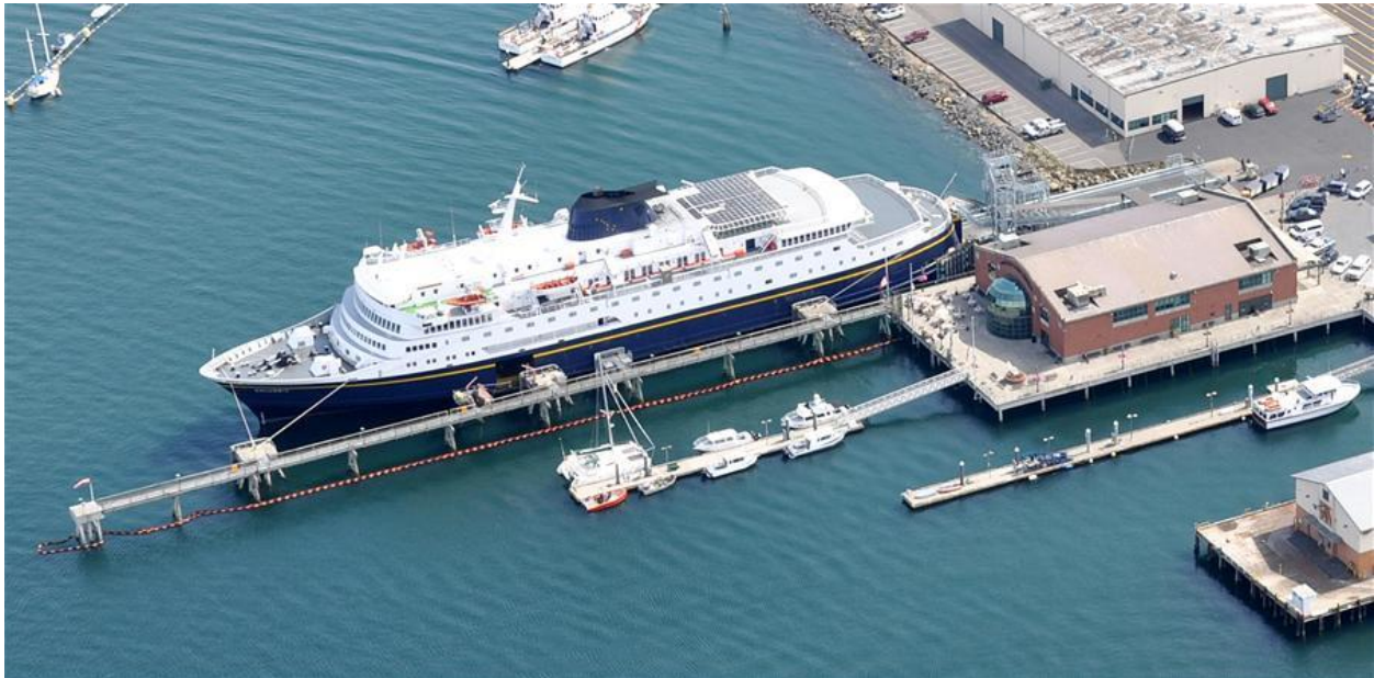
Figure 8: Aerial of the Bellingham Cruise Terminal
