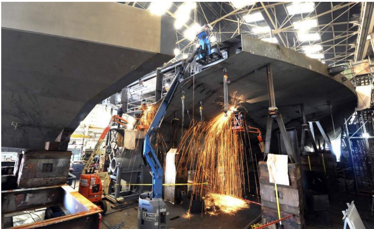
Figure 9, Vigor shipyard workers building a WSF vessel. Photo courtesy of Vigor.
