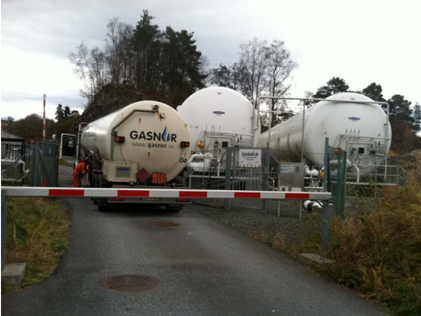
Shore tanks being refueled by tanker truck
