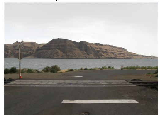
South approach Port Kelley Road, Walla Walla Co.
