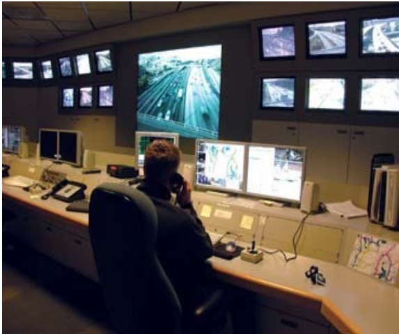
Traffic management center
