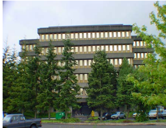
Northwest Region Headquarters
