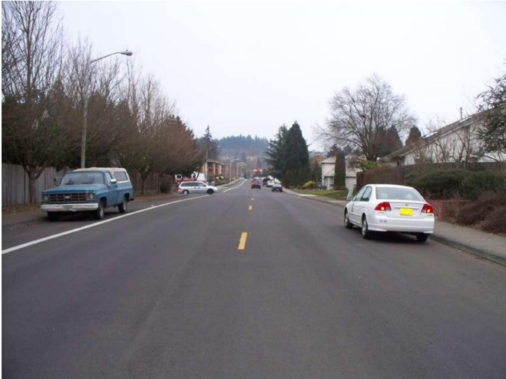
Pavement Condition 93 (Very Good): 108 th Avenue south of Durham Road; Paved in 2007.
