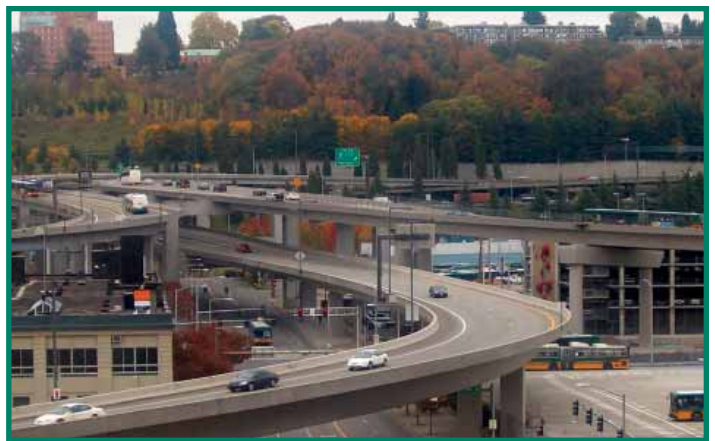
Current 4th Avenue off-ramp from I-90 and South Royal Brougham Way.
