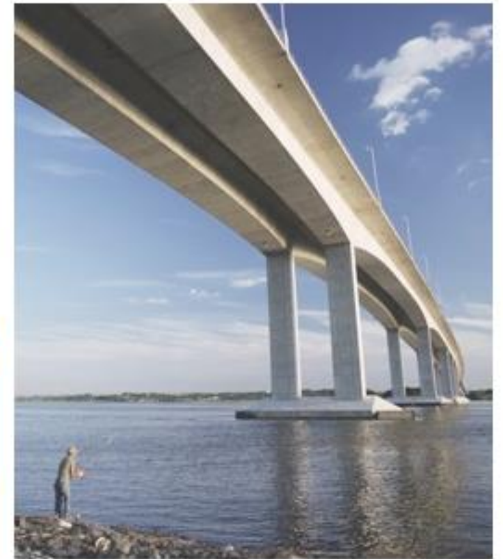
LONG SPAN BRIDGES
