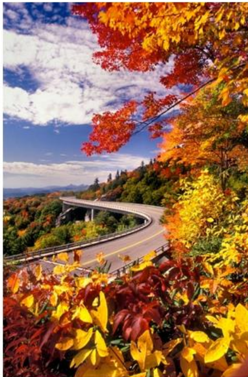
Blue Ridge Parkway Viaduct, NC National Park Service
