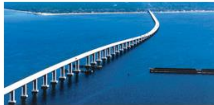
LONG BRIDGES OVER WATER
