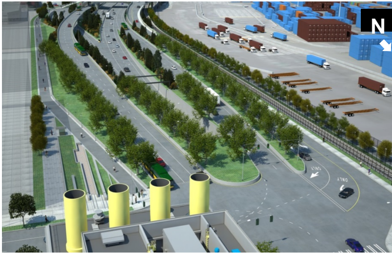
Tunnel connections and surface streets at the south tunnel portal
