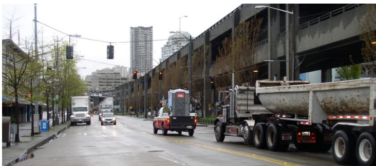
City of Seattle rebuilds Alaskan Way along the waterfront
