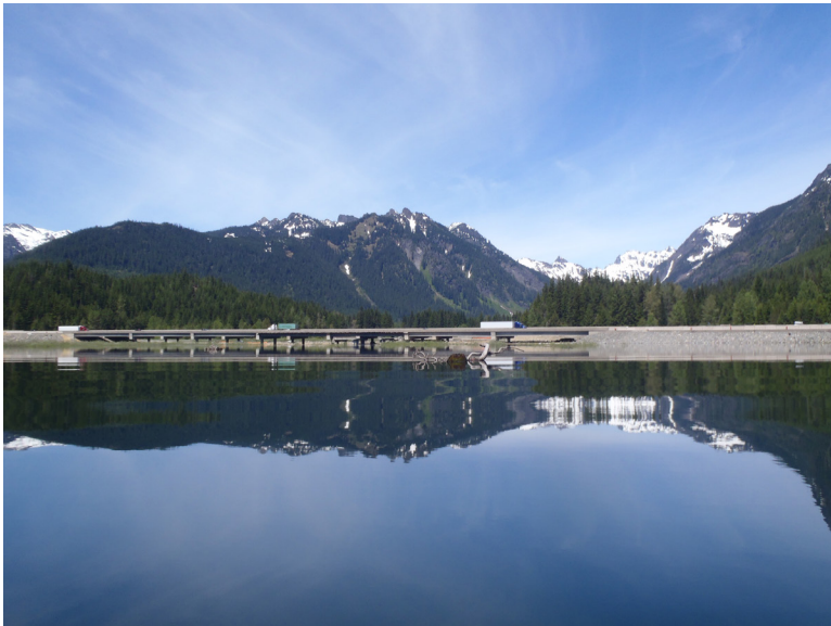
New bridges at Gold Creek (June 2012).
