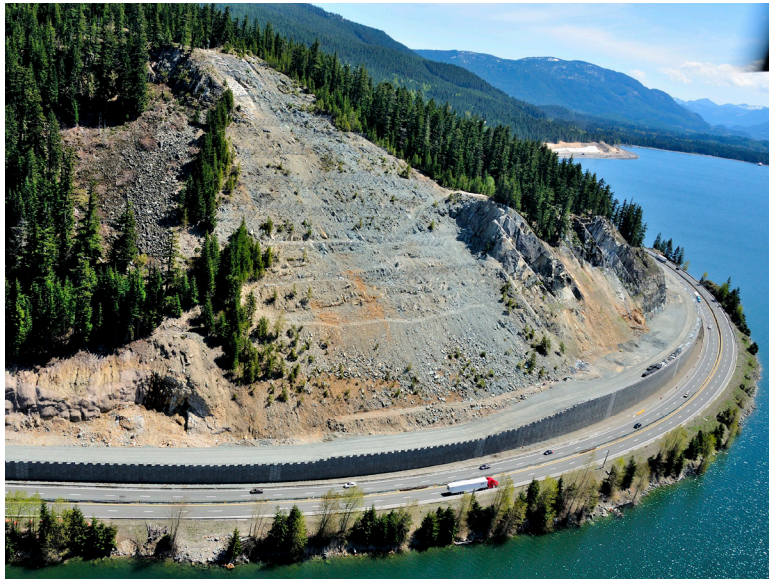
I-90 Slide Curve construction (April 2016)
