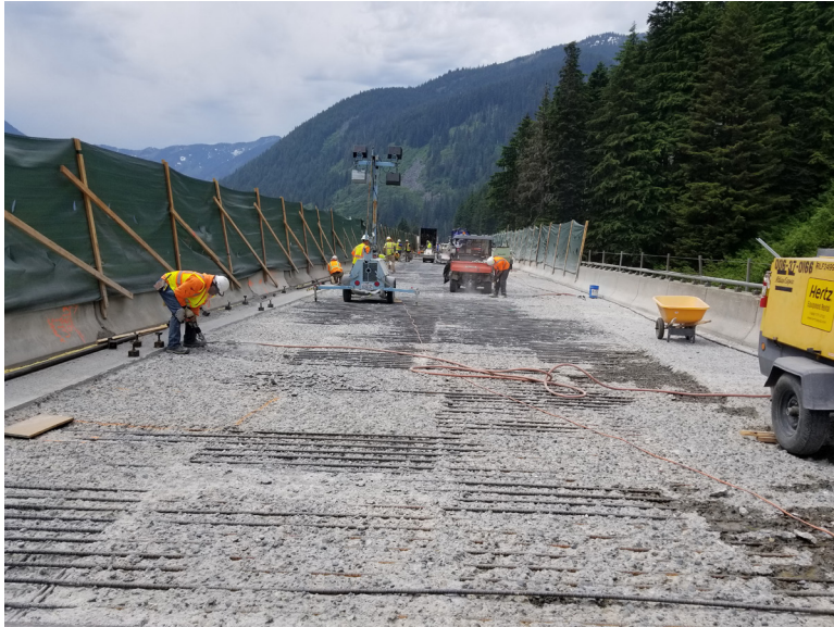
Repairing the I-90 westbound viaduct bridge deck (August 2017)
