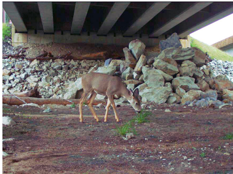
Wildlife crossing under new bridges at Gold Creek (October 2014)
