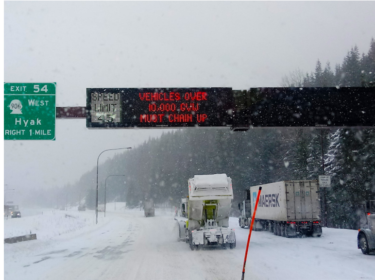
ITS signs and chain-up areas (December 2016)
