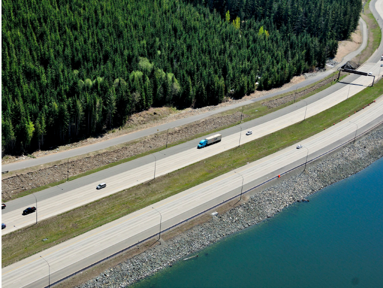
New chain-up area along I-90 (April 2016)
