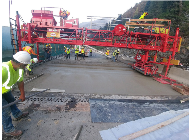
Placing the concrete bridge deck (August 2017)
