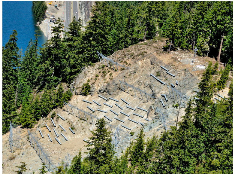
Avalanche Fences constructed at Slide Curve above I-90 (April 2016)
