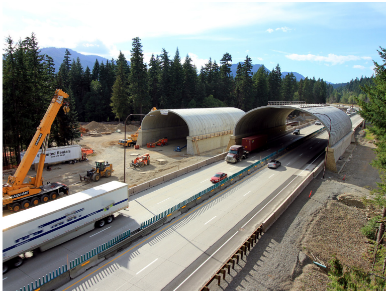
I-90 Price/Nobel Wildlife Overcrossing construction (August 2017)
