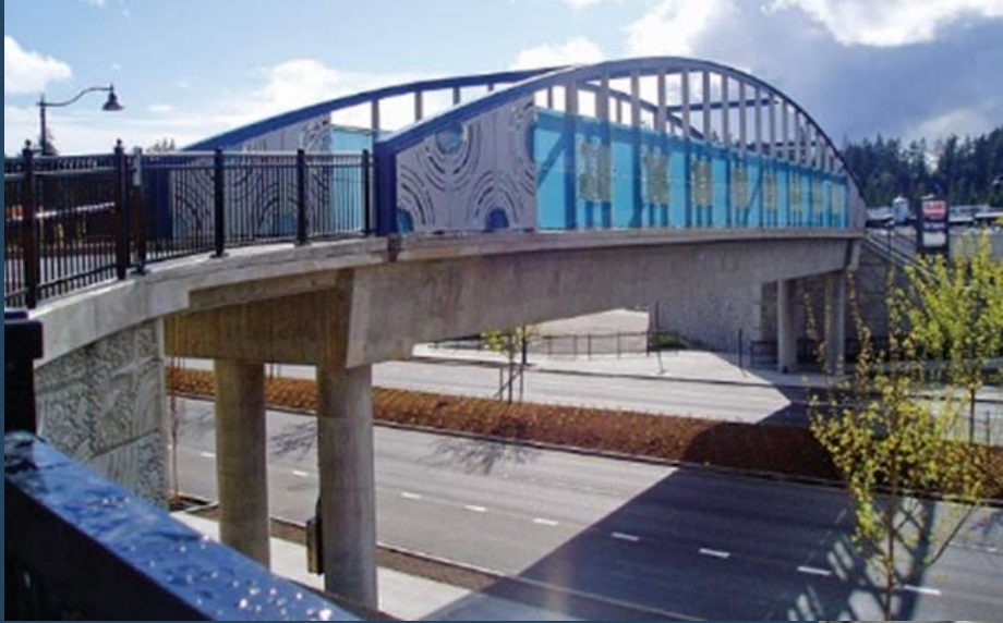
Above Grade Crossing
