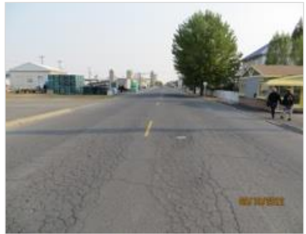
First Street Project. Source: TIB.
