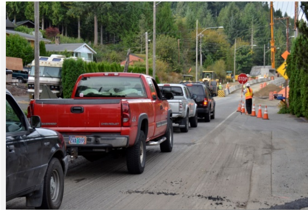
Example of Traffic Control
