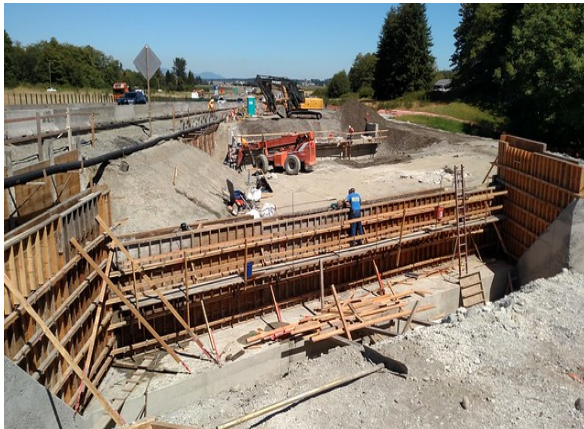
Example of Bridge Construction
