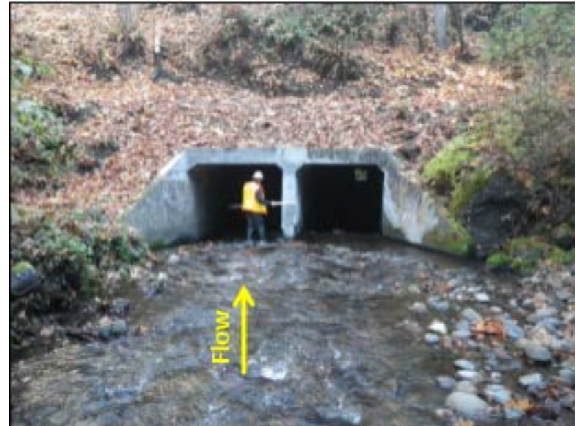
Existing culvert inlet upstream of US101
