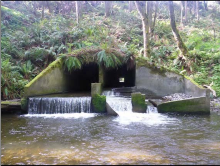
Existing culvert outlet downstream of US101
