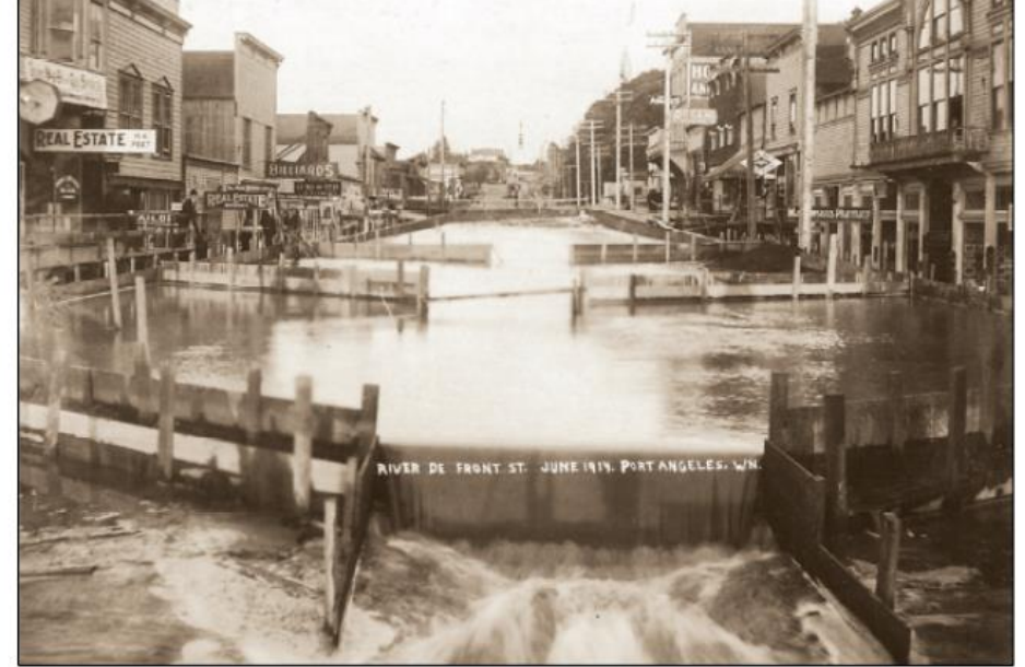
Picture 10: Port Angeles regrading
