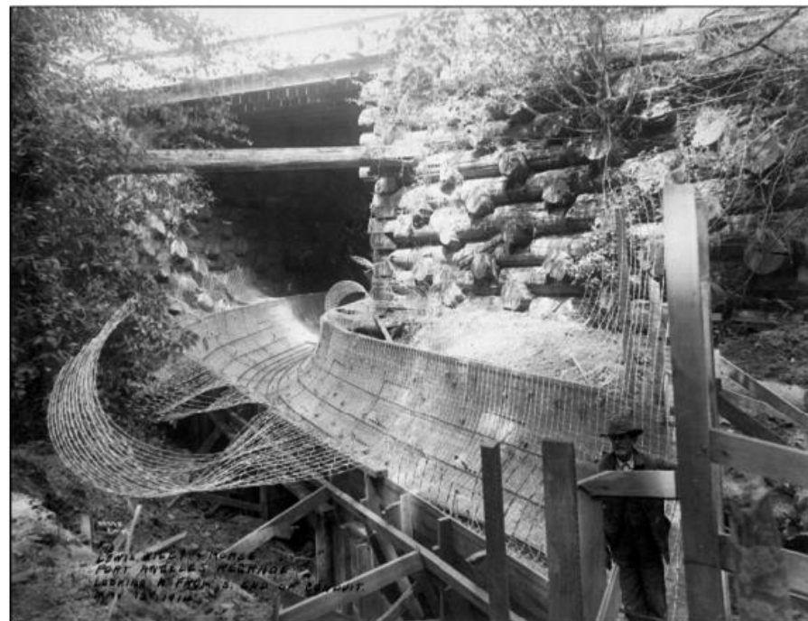
Picture 2: Construction of bend to the north from entrance (looking north)
