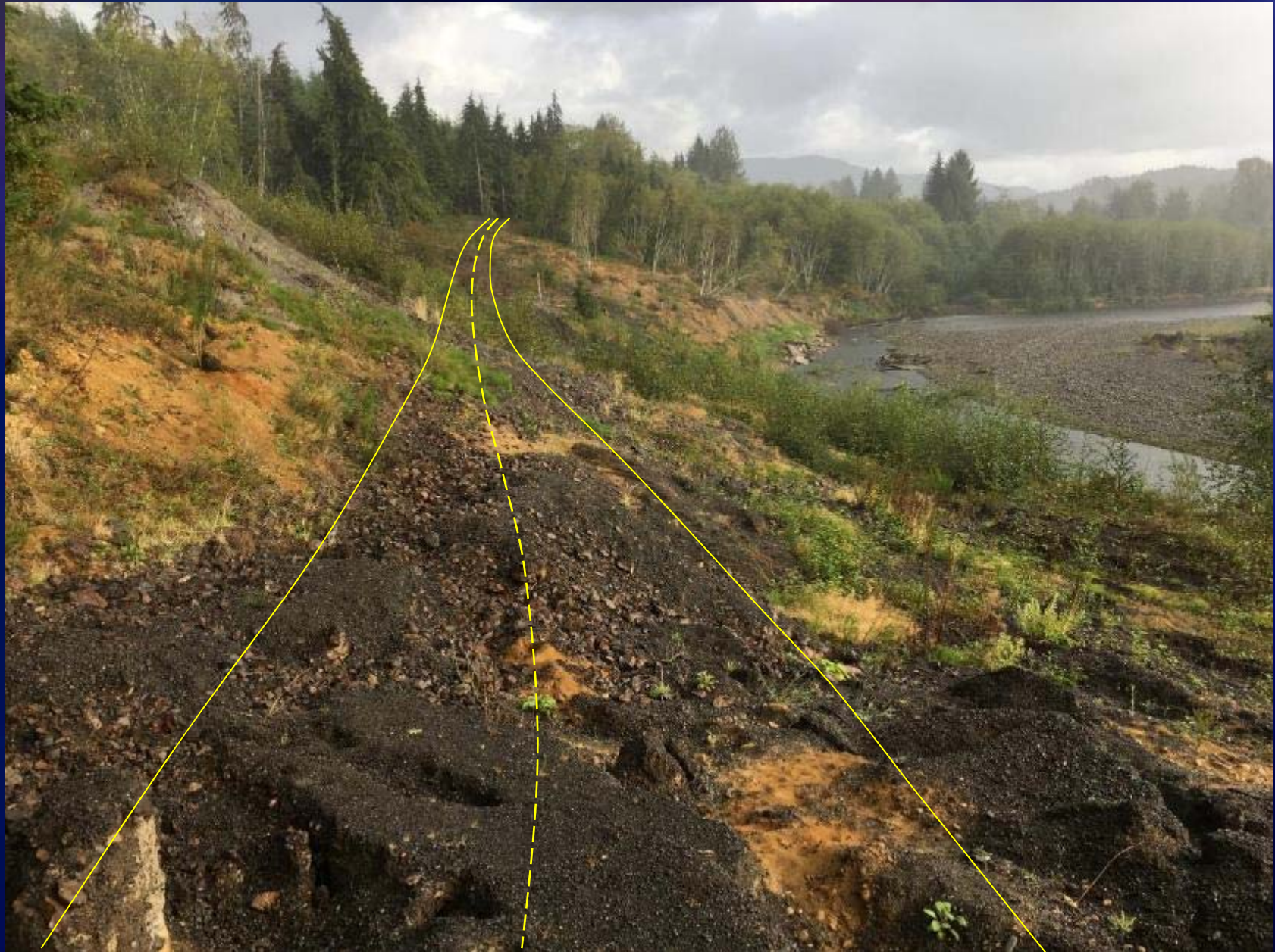
Undi Road – 2016 Landslide Bogachiel River Access to Olympic National Park
