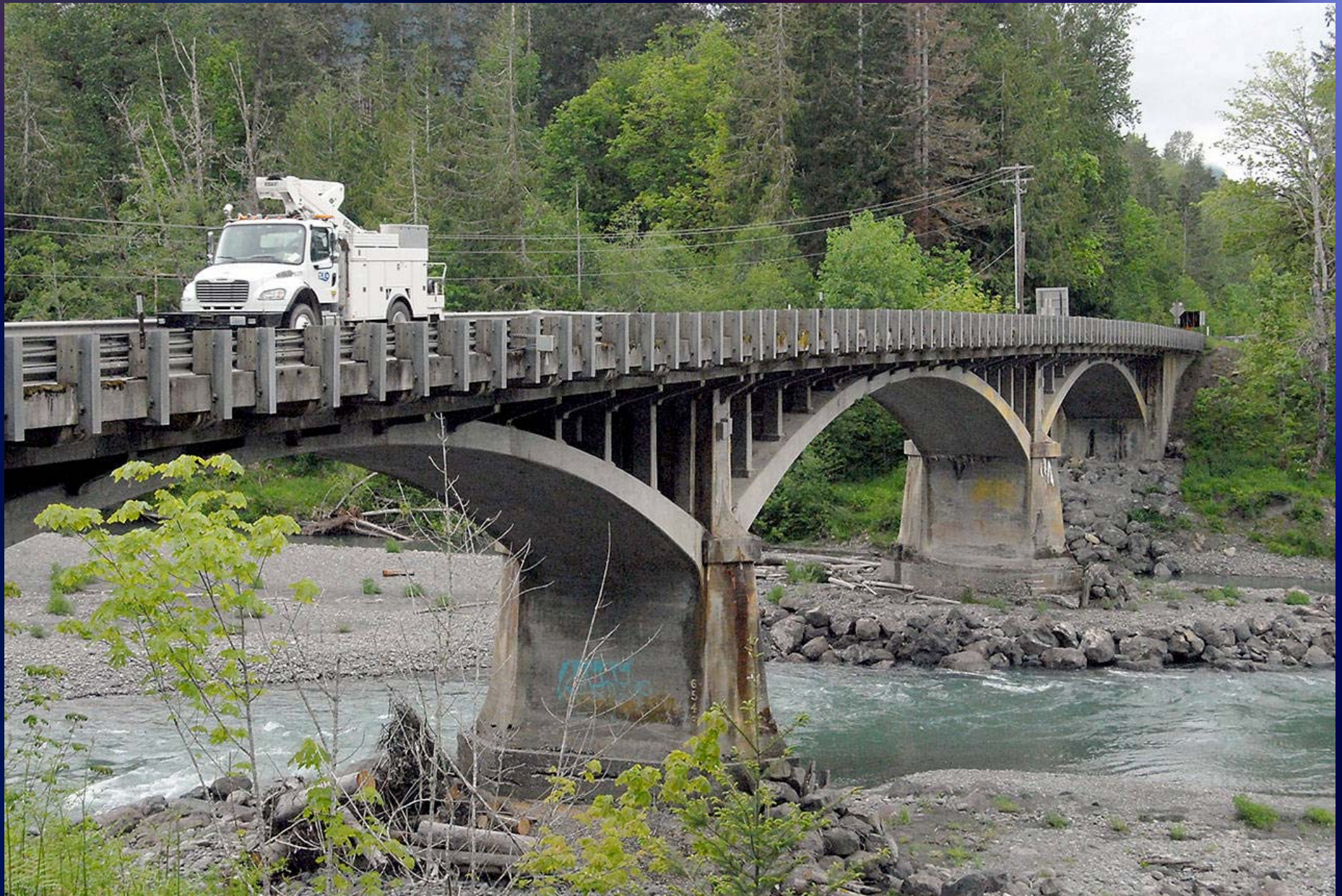
Elwha Bridge (US-101) – The Vital Link to the West End
