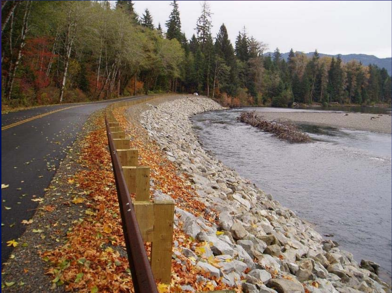
2007 Repair – Jefferson County
