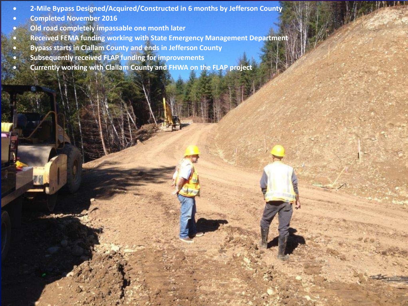
Undi Road – Emergency Bypass (Now permanent)
