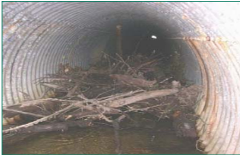
Culvert Plugged with Sediment or Debris
