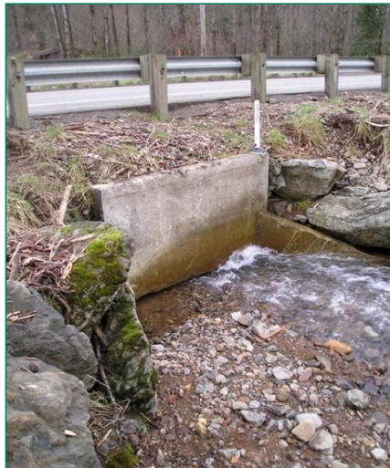
Culvert Plugged with Sediment or Debris
