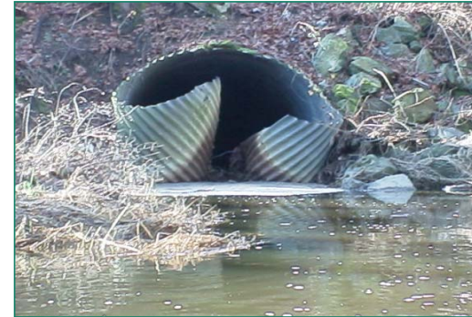
Deteriorating Culverts
