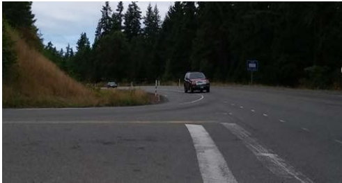
US 101/Palo Alto Road looking west
