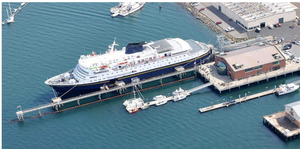
Figure 8: Aerial of the Bellingham Cruise Terminal 38
