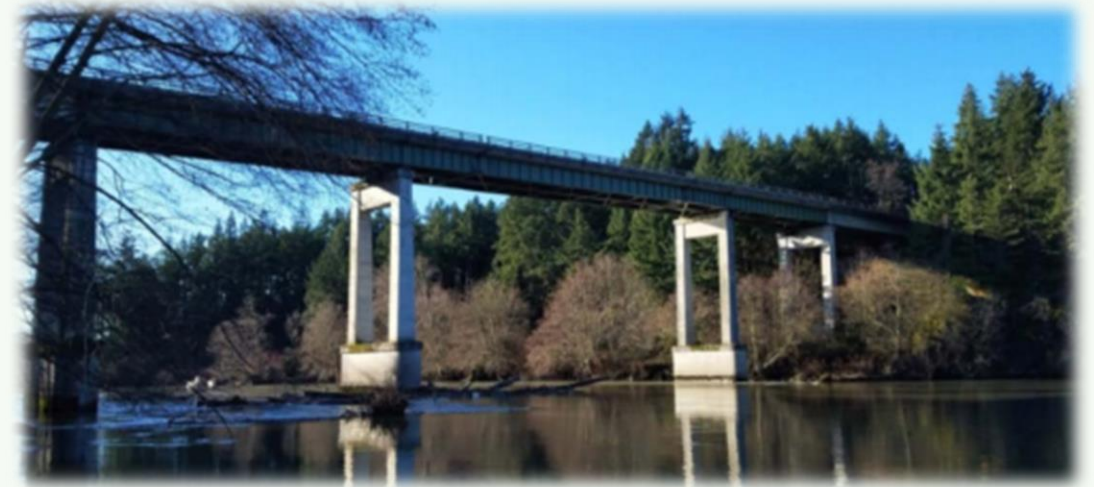
North Fork Bridge
