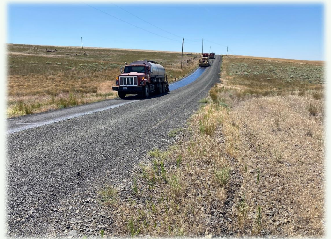
Bituminous Surface Treatment in Progress
