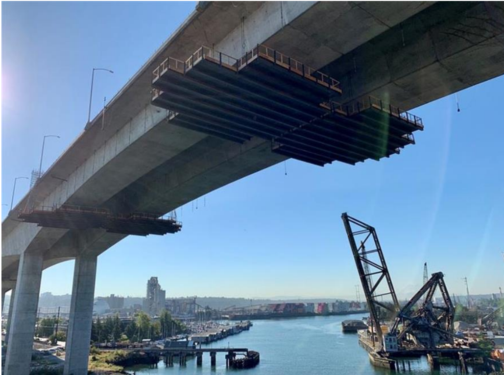
Work platforms installed in July
