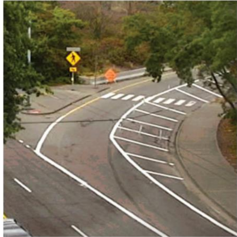
After: ramp reduced to a single-lane entrance with a metered shoulder downstream of the striping
