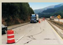
The highway pavement on I-90 is between 30 and 50 years old, and has exceeded its lifespan. Due to extreme weather conditions and heavy usage, the asphalt pavement is rapidly deteriorating.
