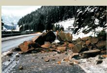
Falling rocks from unstable slopes ranging in size from small stones to complete slope failures have caused serious accidents, and closed traffic lanes.
