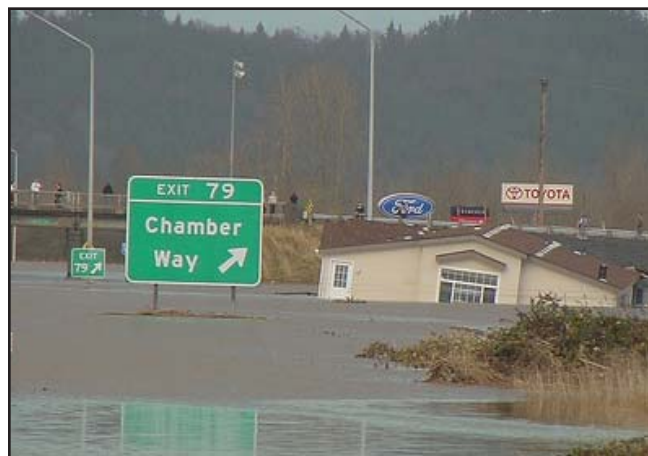
Flooded I-5 Exit 79 in Chehalis
