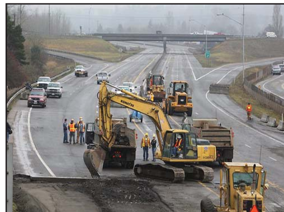
Crews repairing I-5 damage caused by the floods
