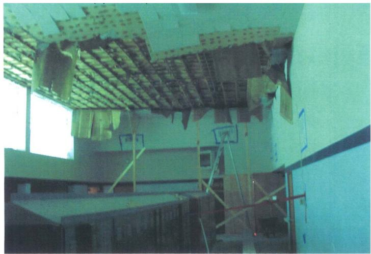
The ceiling of the boys' locker room collapsed between 4 pm and 5 pm, April 2008—but was it anything other than poor construction from the 1950s?
