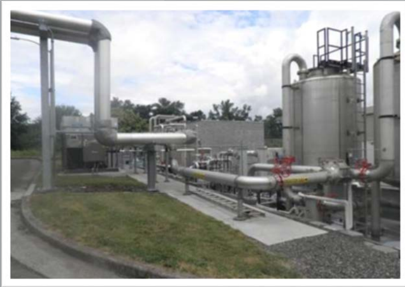
Columbia Blvd waste water treatment facility pipes sending biogas to generator, Portland, OR
