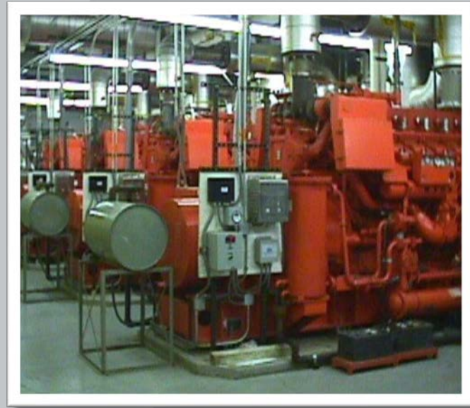
Typical CHP generators
