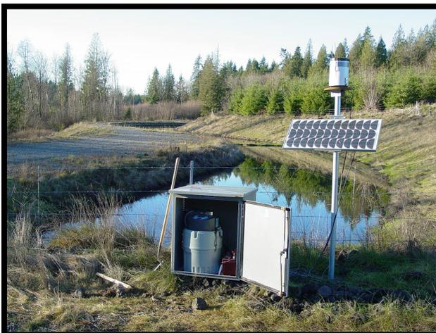
Bioswale and Infiltration Pond – increases natural seepage into the ground
