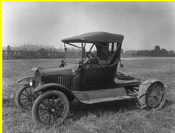
Model T Ford adapted to be a tractor, ca. 1919
