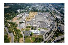
2. Tacoma Central WWTP in Tacoma: Staff in Tacoma note that the plant currently produces RNG that does not meet pipeline grade specifications. In early 2020, Tacoma Central finalized a contract to sell their RNG to Puget Sound Energy. Two steps remain: the plant needs to install equipment to ensure the RNG meets pipeline grade specifications, and a connection must be built between the WWTP and the main natural gas pipeline. The estimated completion for these is June 2021.
