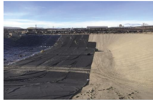
Liner installation for lagoon
