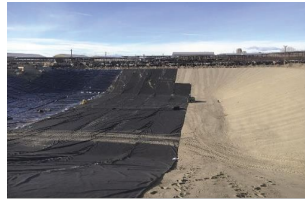
Liner installation for lagoon
