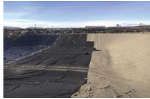
Liner installation for lagoon
