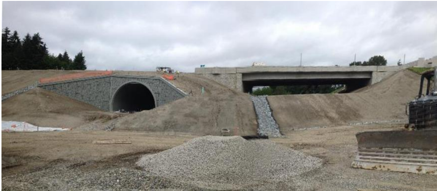
Early Work – City of SeaTac 24 th Avenue
