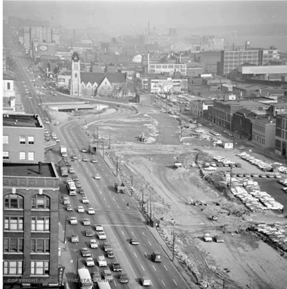
Chrysler Freeway construction in Detroit, MI
