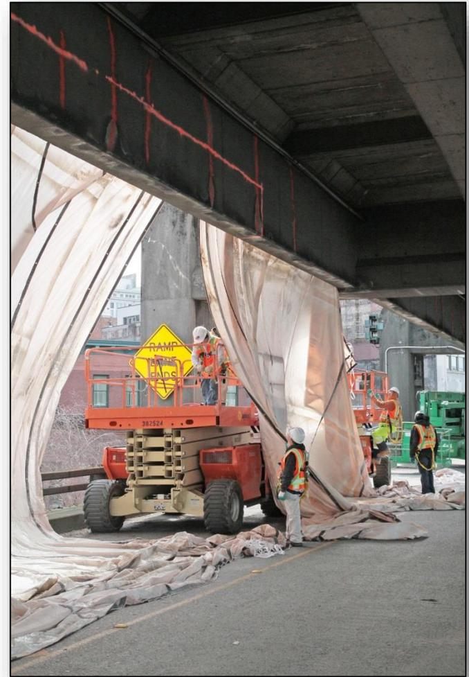
*Crews reinforce the viaduct in 2012 in preparation for the tunneling machine's passage beneath the structure.*
