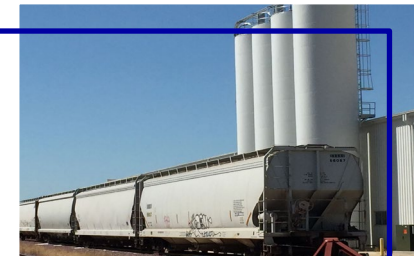
Silo for intermediate handling
