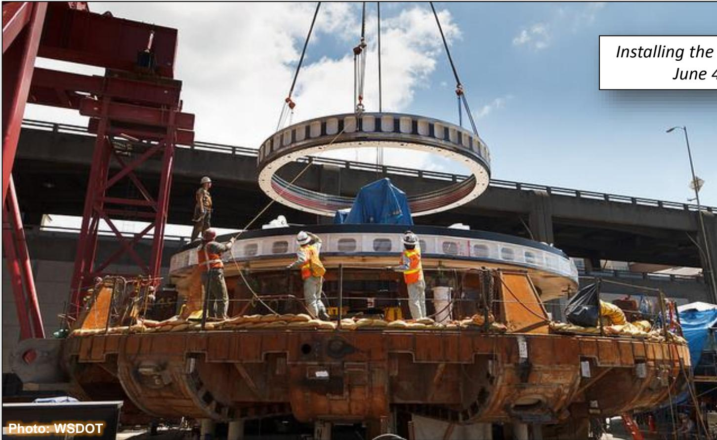
*Installing the inner seal ring
