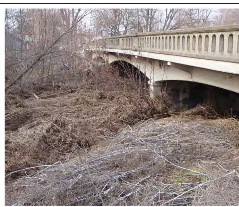
Figure 6. Shows Preston Ave Bridge Facing West, Note the Two Tiers are Full of Brush and Silt, 2/19/09. Photograph by Alex Amonette
