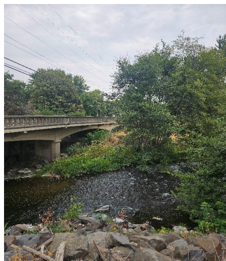
Figure 6. Shows Preston Ave Bridge Facing West, Note the Two Tiers are Full of Brush and Silt, 2/19/09. Photograph by Alex Amonette
