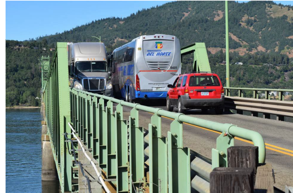
Narrow lanes and shoulders on existing bridge do not meet current standards
