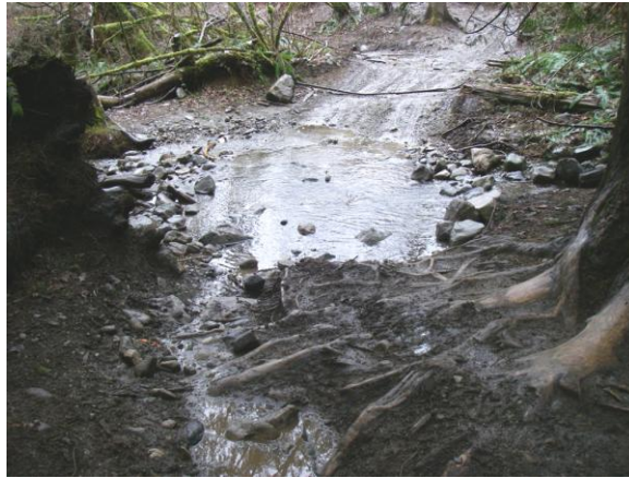
Stream damage at Reiter Foothills Forest
