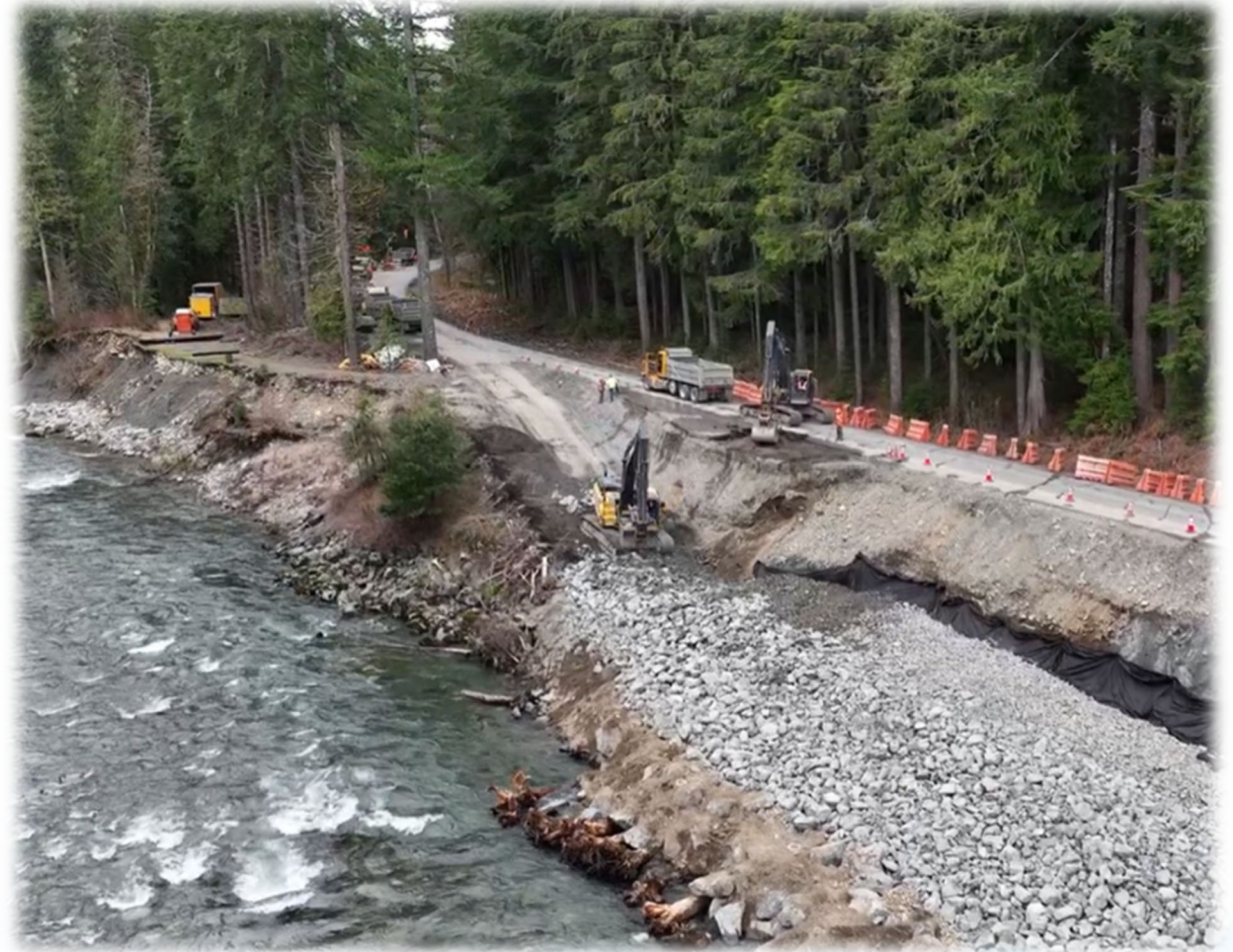
Slide repair at Marten Creek Bridge – Index Galena
